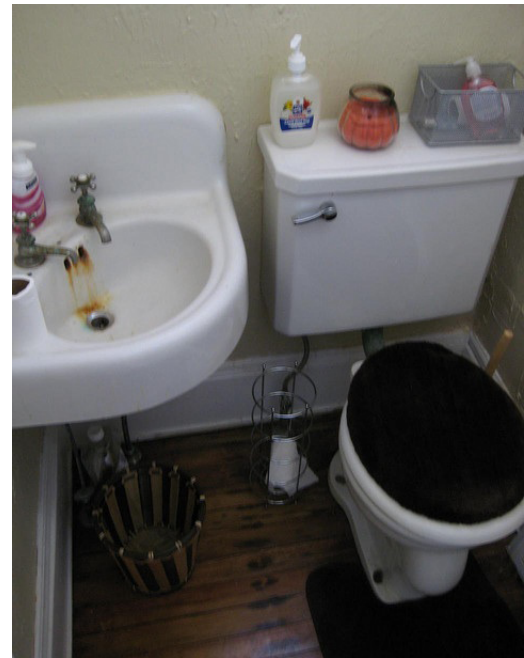
Figure 12: Typical stains caused by iron in water. (Source: smoMashup, Flickr.com)
